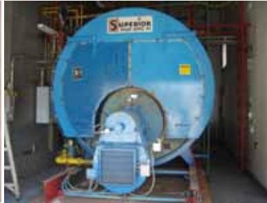
Gas Fired Boiler - 500hp
