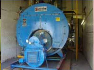
Gas Fired Boiler - 350hp
